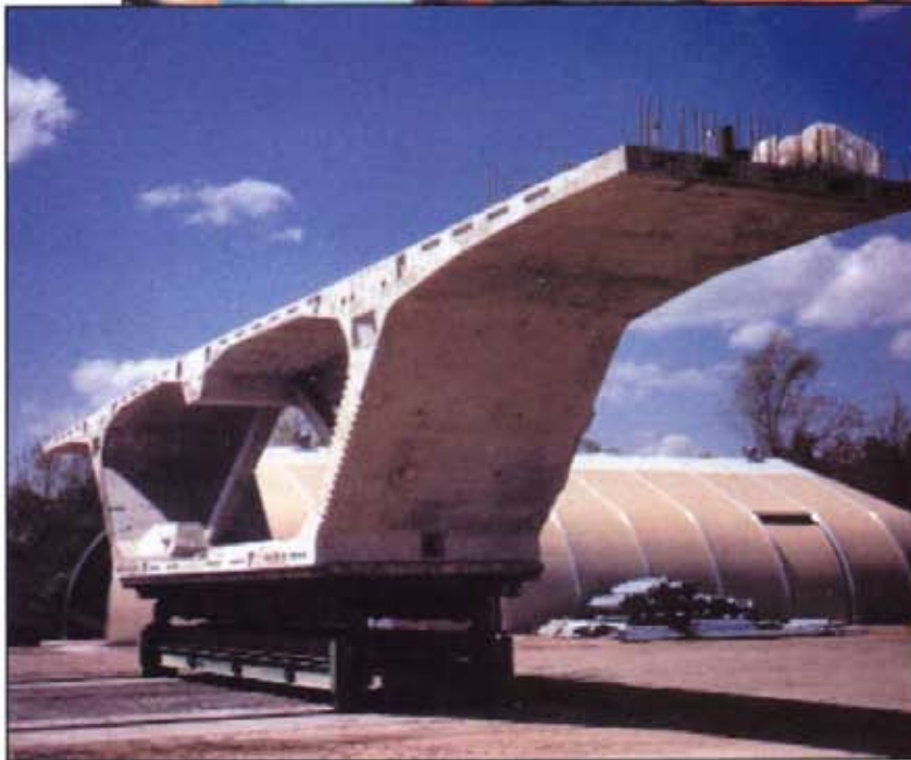
BRIDGE SECTIONS CAST ON SITE
