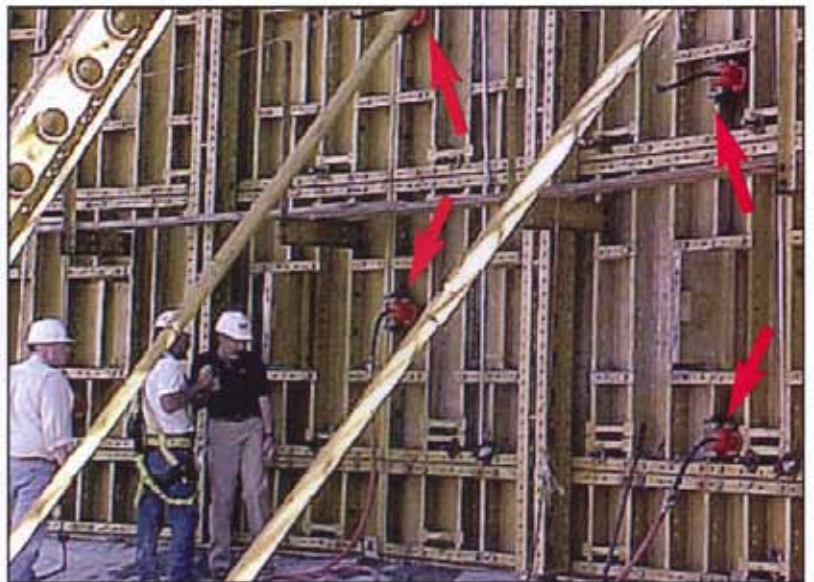
Close up of vibrator spacing.
