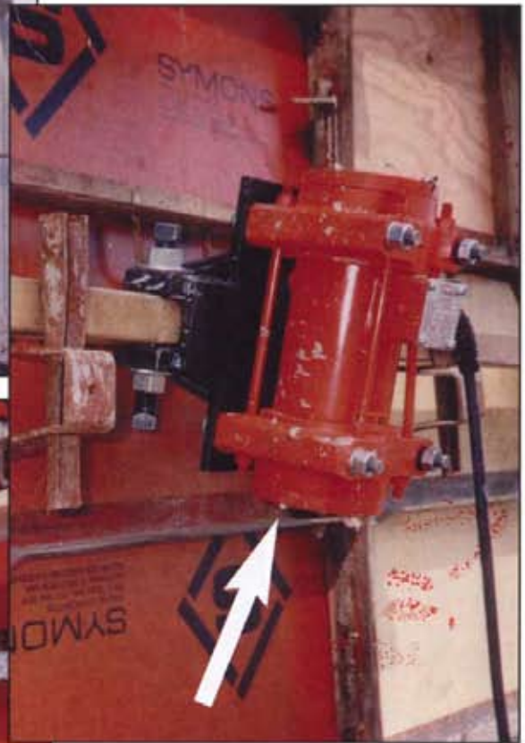
Bracket with vibrator clamped to a 2 x 6.
