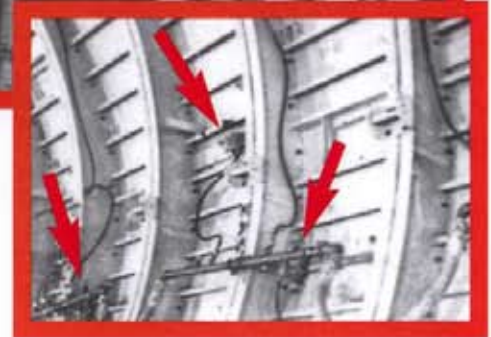
224 VIBCO High Frequency Air Vibrators used in casting New York water tunnel.
