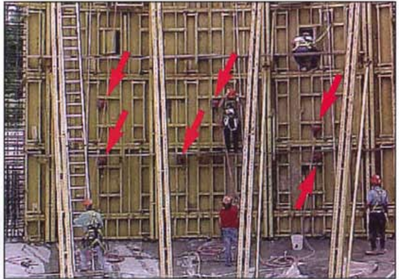
Wall section to be cast – notice the tight rebar.
