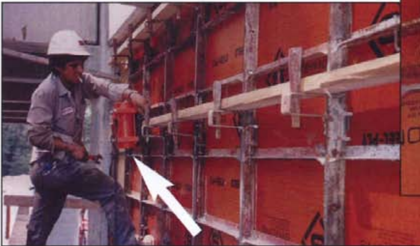
Bracket with vibrator clamped to a 2 x 6.
