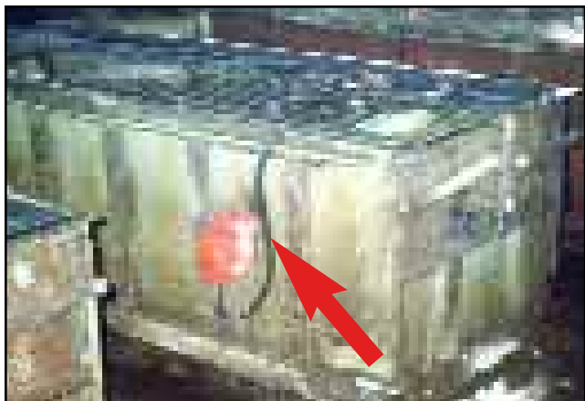
Burial Vault form with VSP-510 Rotary Piston Vibrator.
