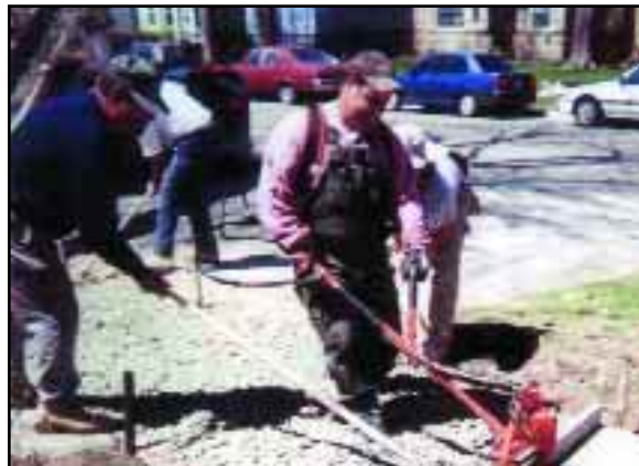
Screed using a 2 x 4 and a pneumatic VS-350 vibrator
