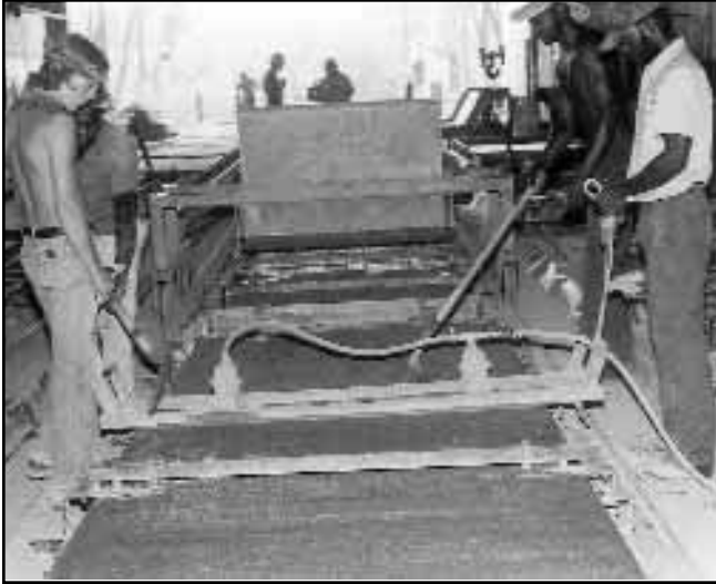
BVS-510FS Turbine Vibrator on 4" screed, made from 4" channel iron.
